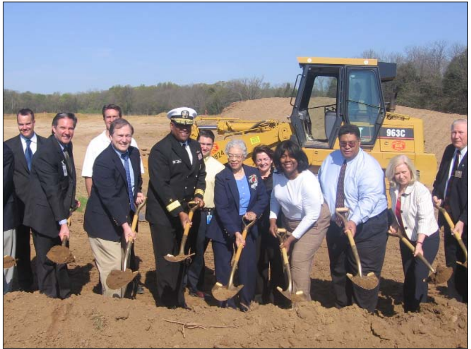
The ceremonial groundbreaking for the Samuel L. Gravely Elementary School attracted members of the Prince William County community and Navy representatives. Among the dignitaries in attendance were Mrs. Alma Gravely, widow of Vice Adm. Samuel L. Gravely, and Rear Adm. Vic Guillory, deputy director of Surface Warfare, both pictured in the center.
